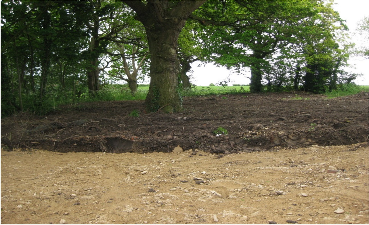
(Above image) 17 May 2018 view of the site observed from roadside at Oldfield Carr Lane. Note evidence of mechanical site scrapping, resulting in key tree disturbed root mass. Foreground displays dug out and stoned up area indicated as for temporary access.
